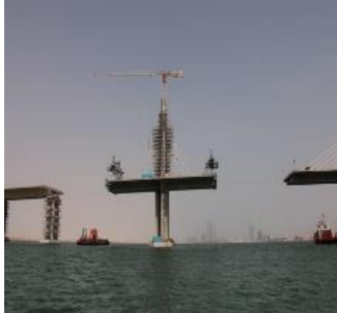
2 nos. TEREX-COMEDIL CTT181-8, H20 at Hodariyat Bridge Projects Abu Dhabi-UAE
