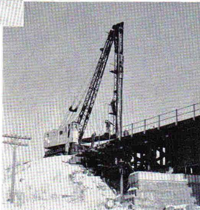
Another elevated cab showing the complete view the operator has to see his work at all times.
