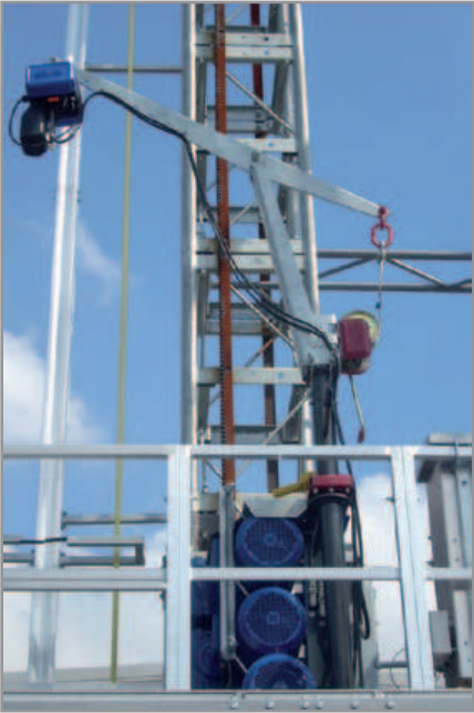
Assembly winch on the cabin roof
