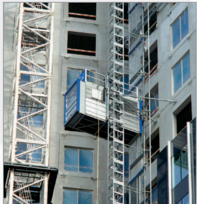
GIANT-Lift 2260FC in operation in Rotterdam
