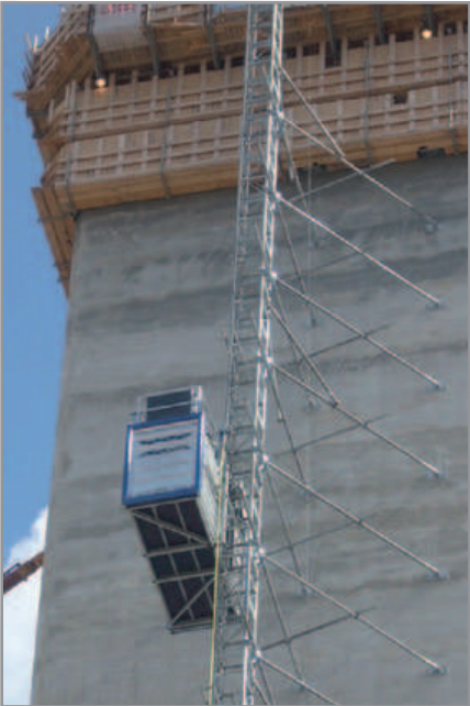
Approach of sliding formwork
