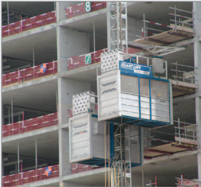
GIANT-Lift 2260FC in operation in Abu Dhabi
