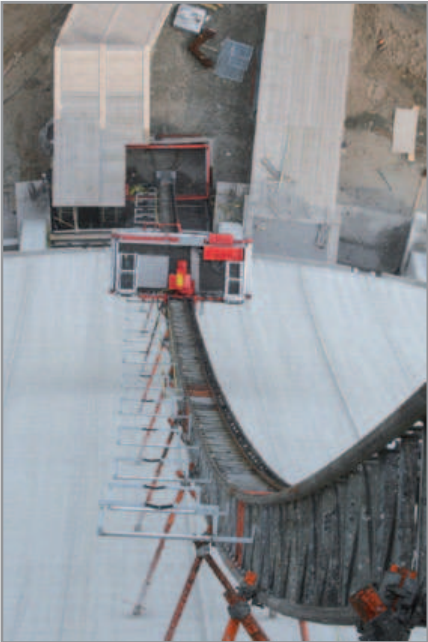
Curved mast for approach of cooling tower during the construction of a power plant
