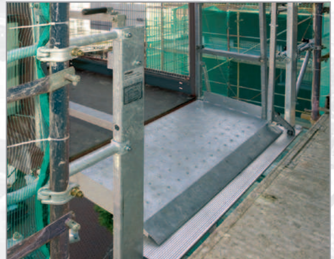
Landing with opened platform ramp
