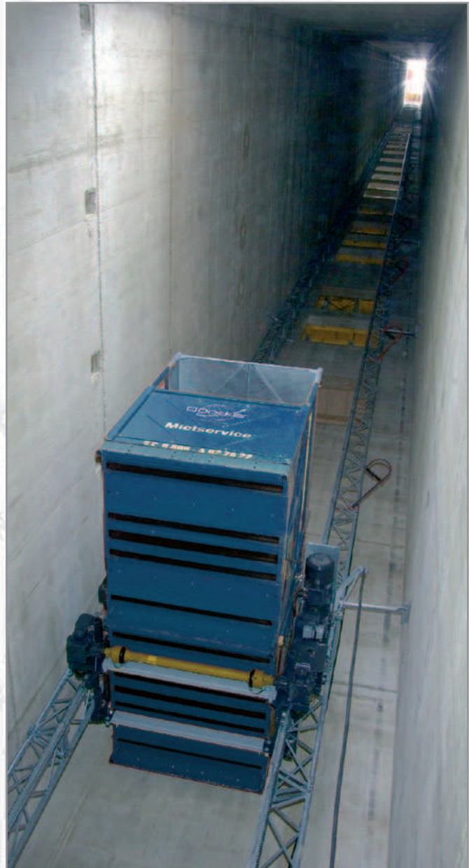
MX 1524-A34 installed in a lift shaft
