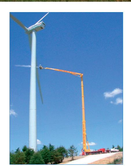
With the Bronto aerial work platform cleaning the blades can be done safely and effectively.
