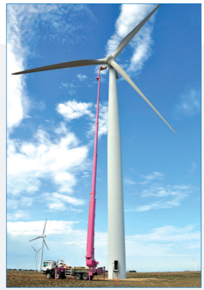
XDT unit gets the work done.
