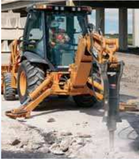
Optimized hose routing for demolition work
