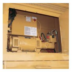
**Generator Set.** A 20 kW hydraulically driven generator set can power magnets of 66" (1676 mm) in diameter. A Baldor generator and electronic magnet controller manufactured by Cat are linked to provide trouble free service. This controller virtually eliminates traditional contractor maintenance.
