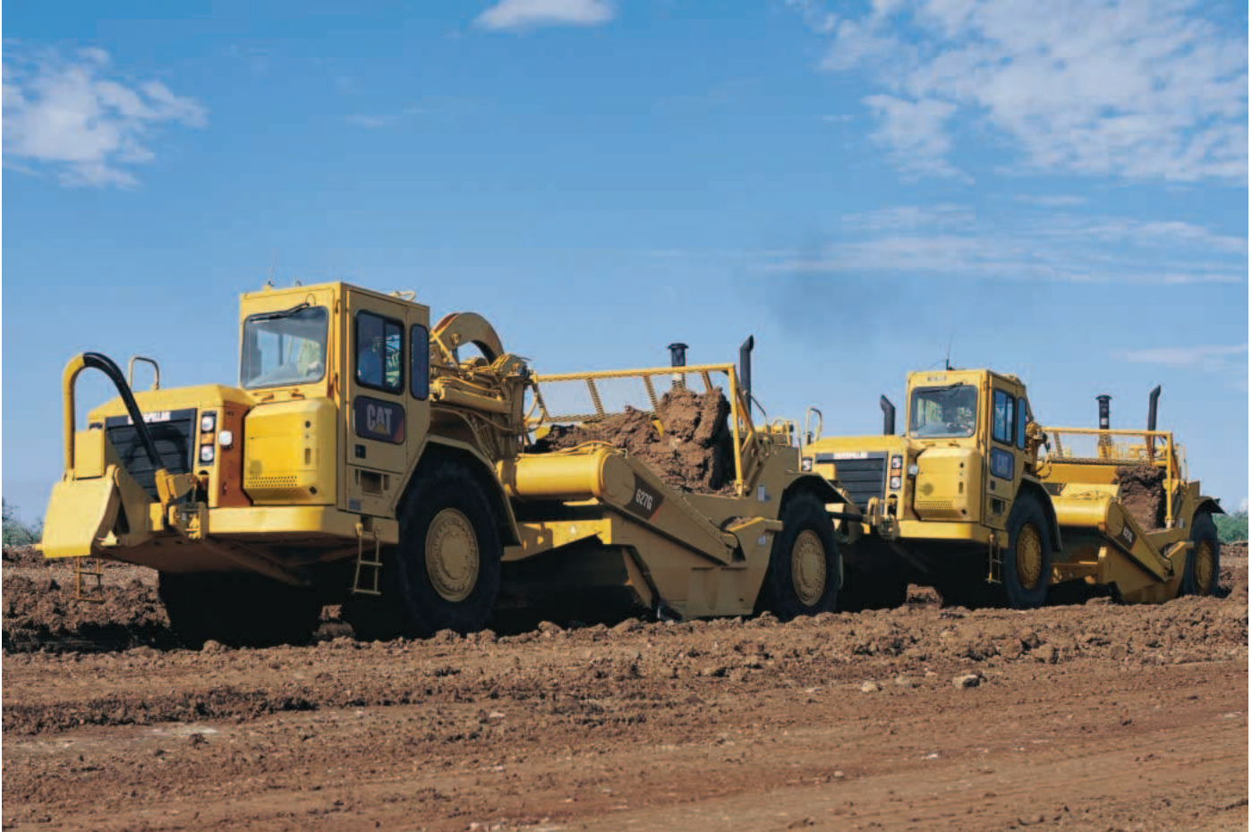
Typical push-pull operation using twin 627G machines.
