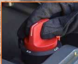
Battery cut-off switch
