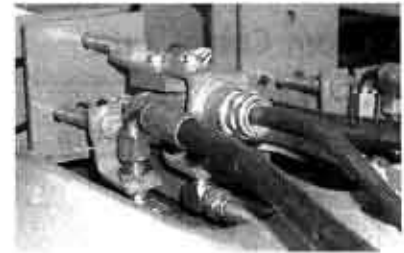
AUXILIARY HYDRAULIC AND ELECTRIC CONNECTION
