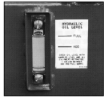
HYDRAULIC OIL LEVEL SIGHT GAUGE
