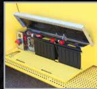
Battery box with Quick Disconnect Switch.
