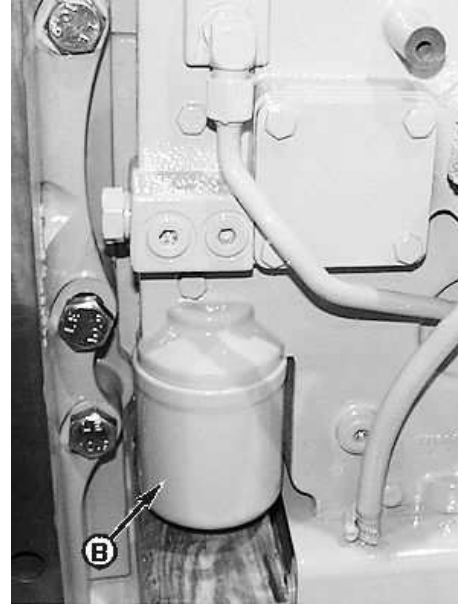
Winch Shown Removed for Clarity of Photo
