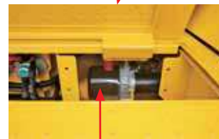
Pump and motor
