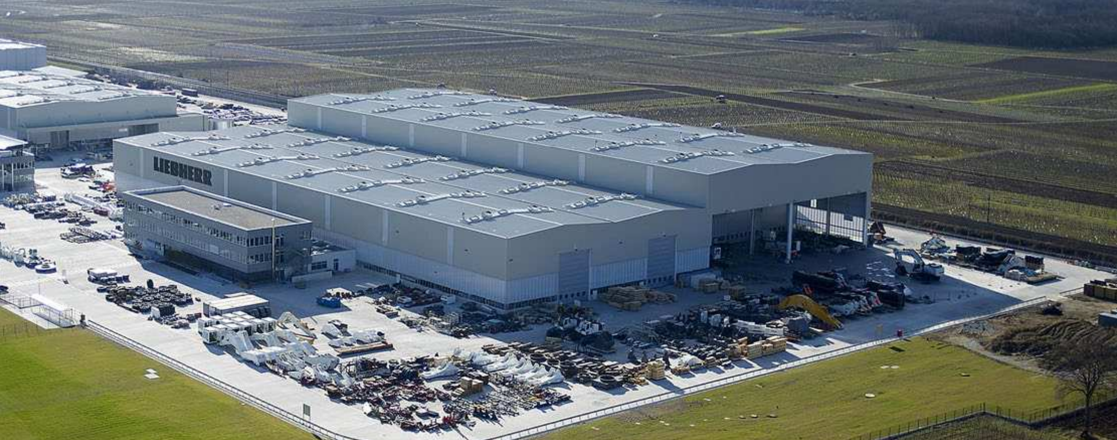
Liebherr-Mining Equipment Colmar SAS, France
