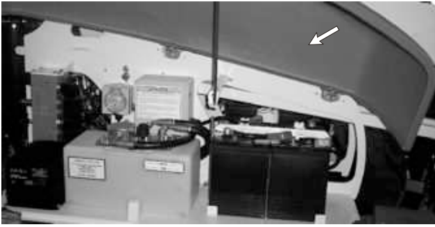
Figure 11.5 - Covers Raised During Charging
