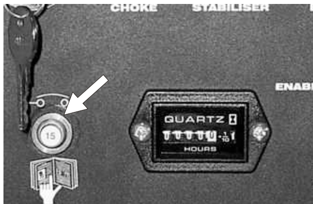
Figure 5.2 - Main Circuit Breaker
