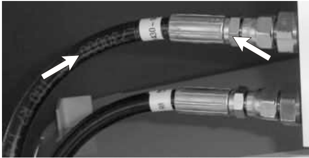
Figure 7.12 - Hydraulic Oil Leaks At Fittings And Hoses
