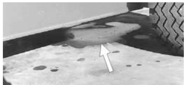
Figure 7.11 - Hydraulic Oil Leaks
