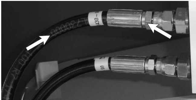
Figure 7.12 - Hydraulic Oil Leaks At Fittings And Hoses
