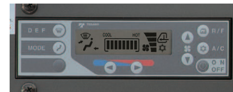
Air conditioning and heating.
