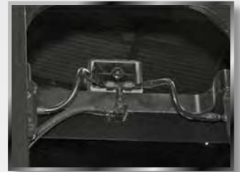
Forward activated alarm
