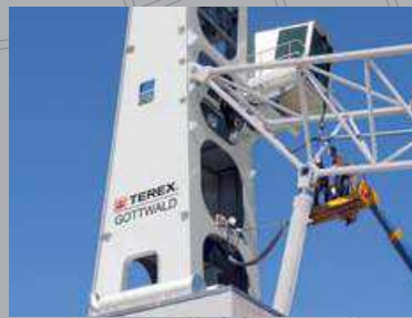
Installation and commissioning
