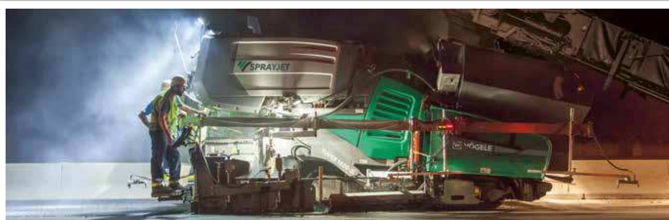
RESURFACING WORK ON A MOTORWAY
