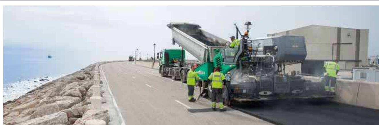
PAVEMENT REHABILITATION OF A CAUSEWAY
