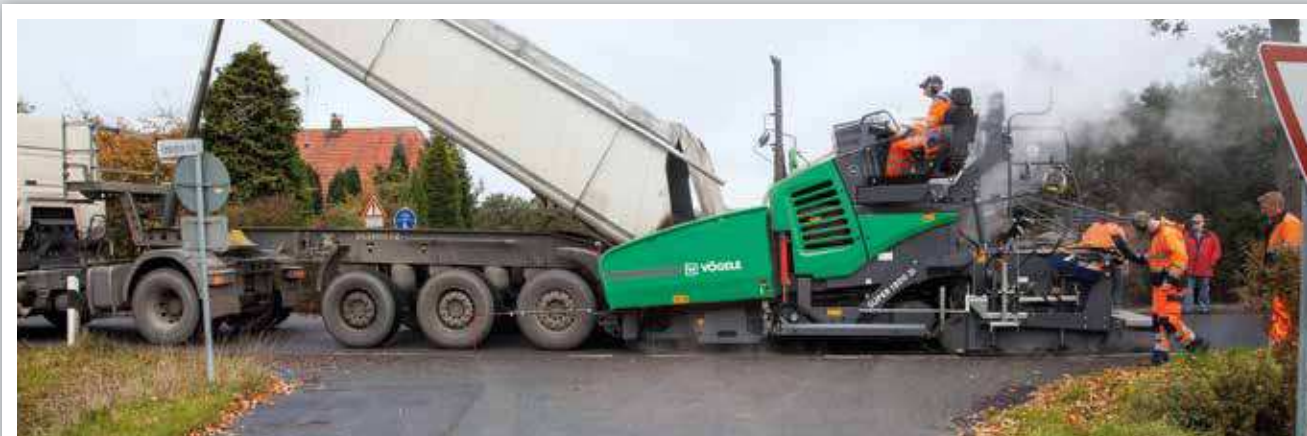
RESURFACING A ROADWAY IN A RESIDENTIAL AREA
