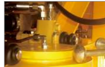
Hydraulic limit system
